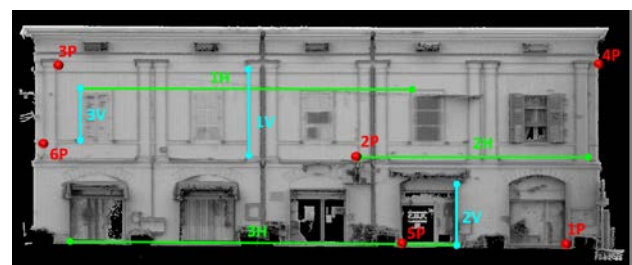
Figure 9. Elements chosen on the Guerrini-Forti palace façade, used for the comparison between the photogrammetric and the TLS model.
