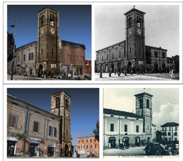
Figure 8. The 3D model of the tower inserted in the TLS cloud of the current context (on the left), from the same viewpoints and in comparison with some historical images (on the right). Upper images: Eastern view; lower images: Southern view.
