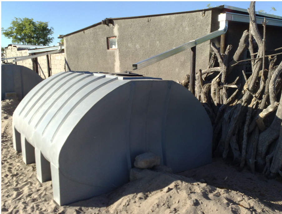
Figure 3.6 Rainwater harvesting pilot plant using polyethylene tanks in the village of Epyeshona, Okatana constituency, approximately 5 km north of Oshakati
