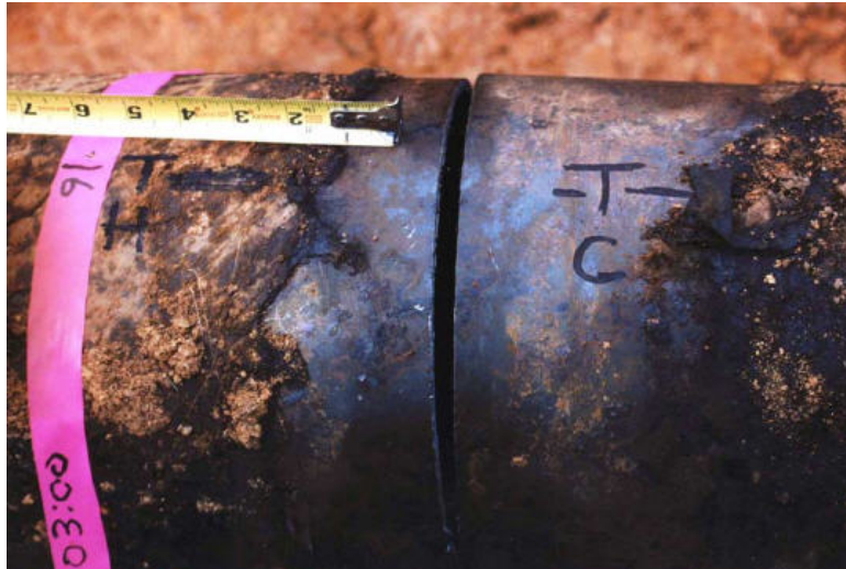
Figure 2.9: Broken metal pipe with 160mm diameter
