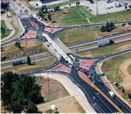
FIGURE 1: Diverging diamond interchange in Springfield, Missouri.
