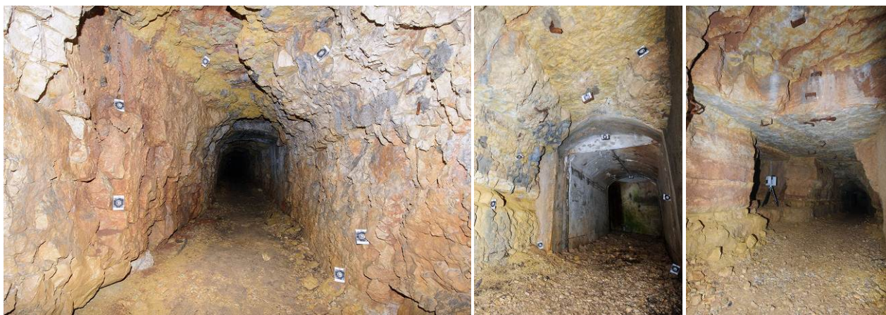
Figure 2. The tunnel - connecting the Viaz and Oberwiesen outposts of the Lusern fortification - with the topographic targets (left and middle) and a TLS station (right).
