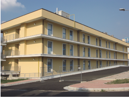
FIGURE 1: View of the hospital building after retrofit.
