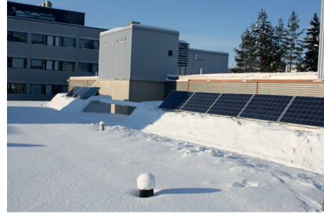
FIGURE 1: Example of partial shading of a PV string due to a building structure on a sunny day during spring 2012.
