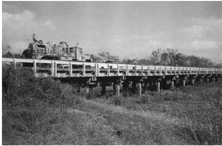
FIGURE 14: Example bridge in Texas.
