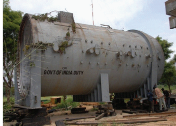
FIGURE 11: Erection of the shell at the site.
