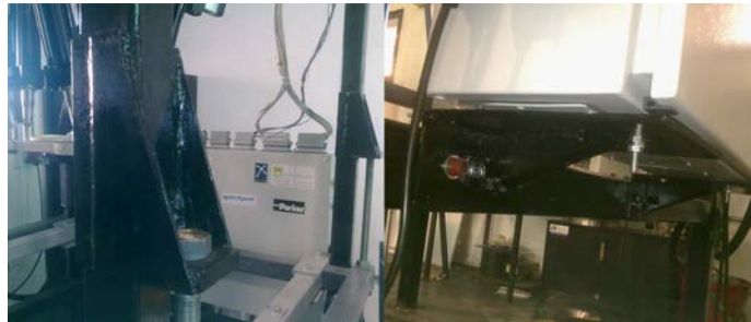
Figure 3.5: Forming table stiffeners and electrical cabinet supports.
