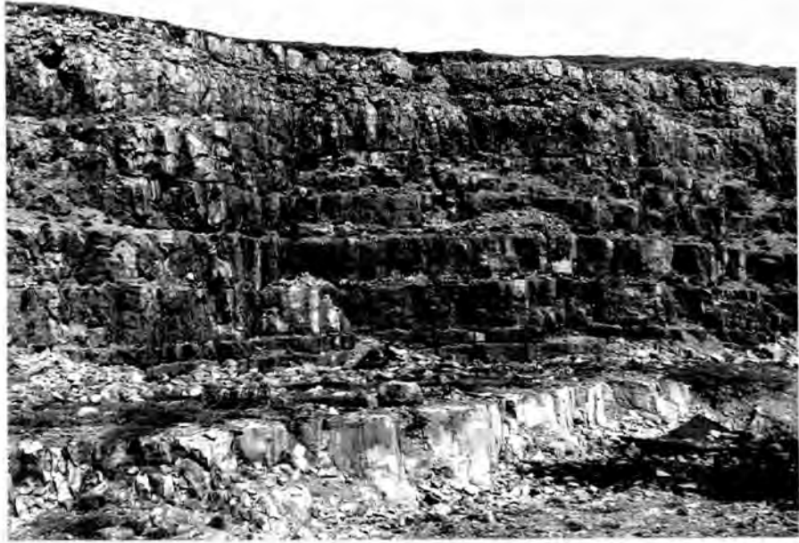
PLATE 35. Even-bedded limestone: the Maulds Meaburn Limestone at Raise Howe Quarry.
