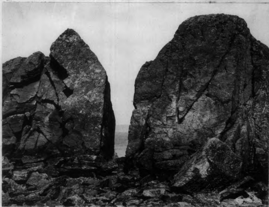
Plate 5.12 PRIMARY AND SECONDARY WRENCH-JOINTS North side of West Angle Bay (9002) Eroded gap is a fault. The primary joints dip left (west) or are vertical, the secondary joints dip to the right. Lower Old Red Sandstone.
