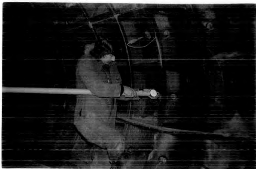
Figure 53 Measuring of the tunnel diameter changes
