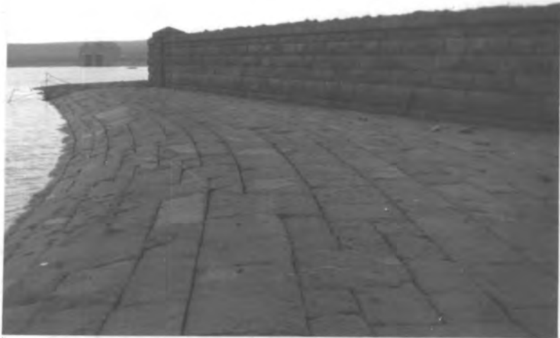
Photograph.4. View from F-10 towards E130,2.5.57.
