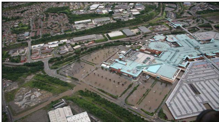
Figure 3. Meadowhall under siege from floodwaters (Image from Peter Smith, 2010)
