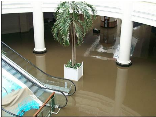
Figure 5. Flooded escalators at Meadowhall (Image from BBC South Yorkshire, 2010)
