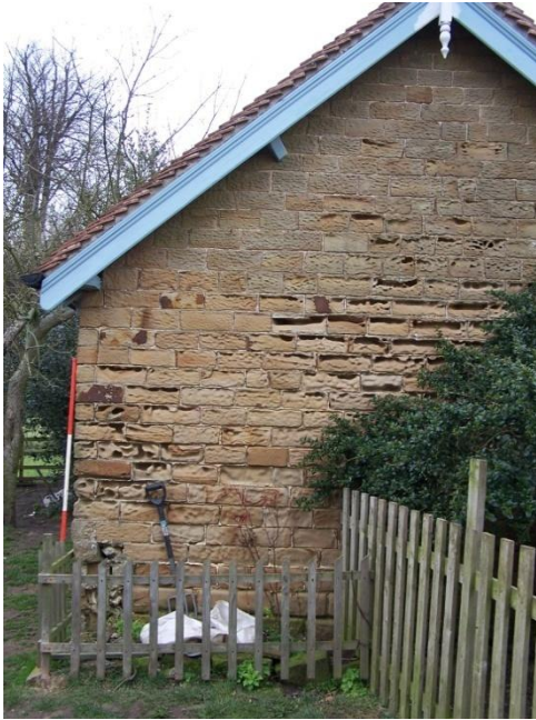
Figure 2: View of southern elevation Norwood Piggeries
