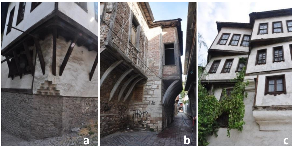
Figure 3: Braced projections from (a) Safranbolu, Turkey and (b) Chalkis, Greece (this concave variation is known as eliböğünde ), and (c) simple cantilever projection from Safranbolu
