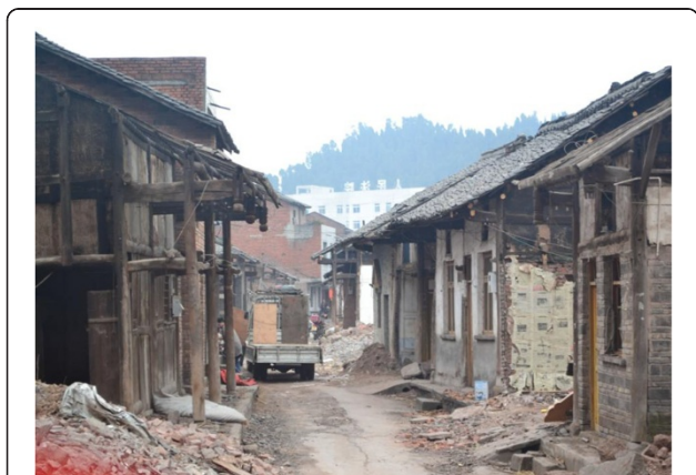
Figure 1 Collapsed houses in Guangyuan after the earthquake.
