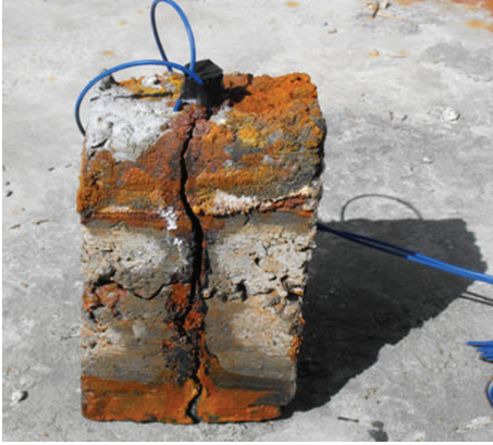
FIGURE 7: Cracking of concrete block.
