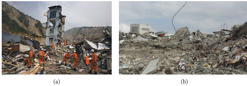
FIGURE 1: (a) Rescue workers searching for survivors after a major earthquake struck Sichuan [17]. (b) Complete destruction of concrete building in Haiti (photo: R. DesRoches) [18].
