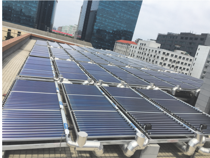
FIGURE 2: Photograph of evacuated tube solar collector with CPC reflectors.
