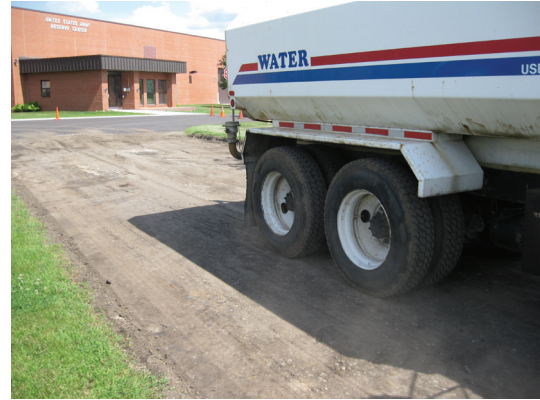
FIGURE 2: Photo showing typical proof rolling test.
