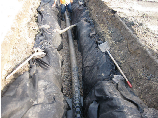
FIGURE 5: Photo showing installation of underdrains.
