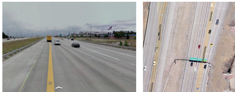
FIGURE 2: A typical diverging area at an off ramp along highway I-25.
