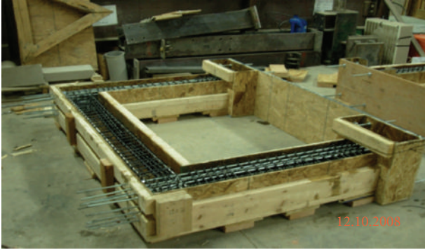
FIGURE 8: Formwork before pouring of concrete.
