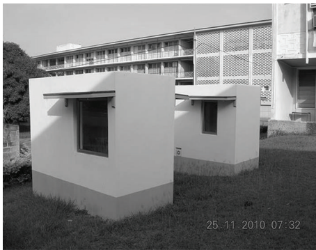
FIGURE 4: Test cells with installations.
