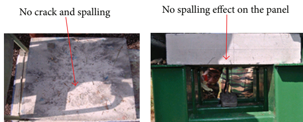
FIGURE 8: Failure mode of HSFRC panel subjected to blast loading.
