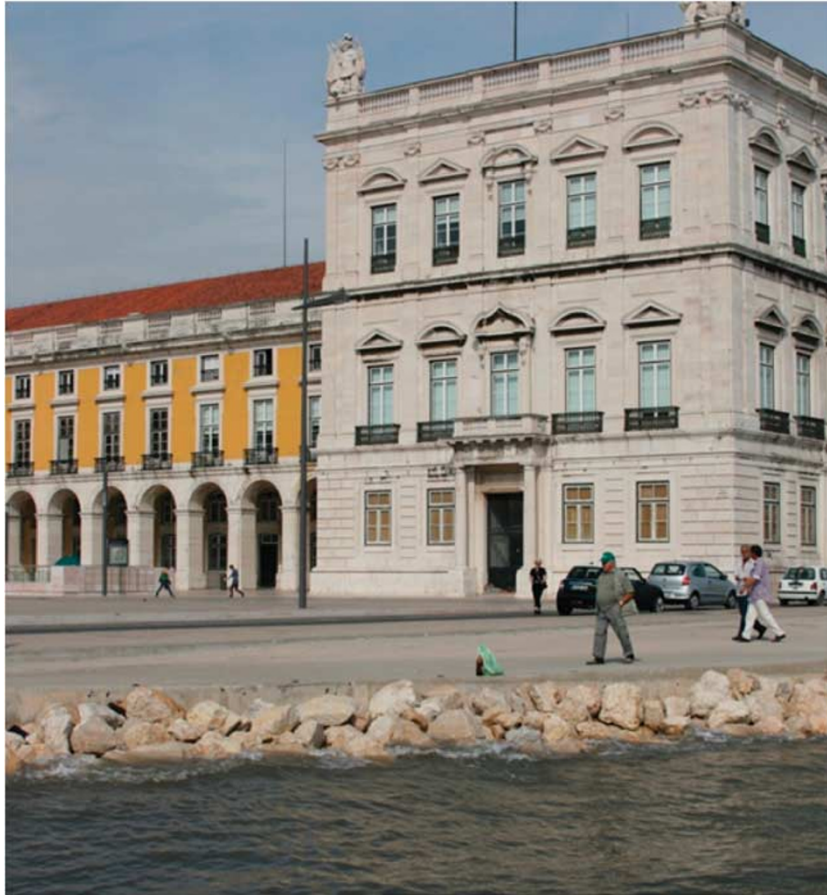
Figure 2: View of Terreiro do Paço during a high tide of 4.26 m. Source: FCT Project 'Urbanized Estuaries and Deltas', FA/UTL and FSHS/UNL, 2011.
