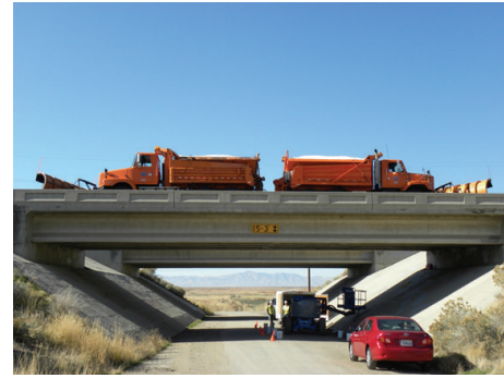
FIGURE 1: Perry Bridge (structure number 1F 205) elevation view during testing.
