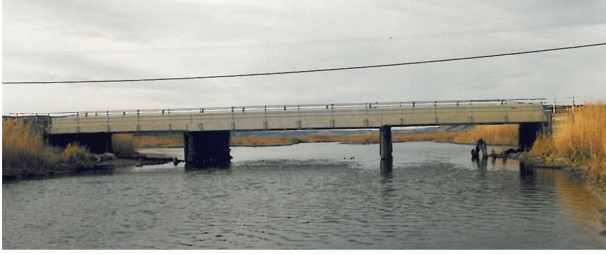
FIGURE 1: Photograph of the bridge prior to girder replacement.
