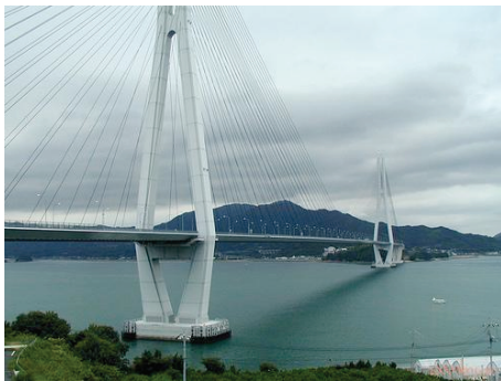
FIGURE 3: Tataru cable-stayed bridge.
