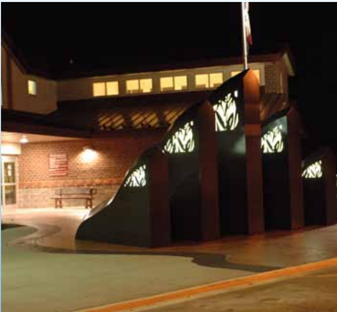
Underwood rest area featuring Loess Hills theme, which is reflected in the backlit columns located in front of the main entrance
