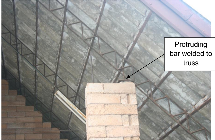
Figure 15: Steel bearing plate with protruding bar welded to roof truss
