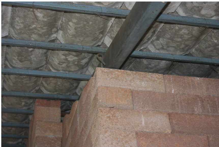
Figure 15: Steel bearing plate with protruding bar welded to roof truss
