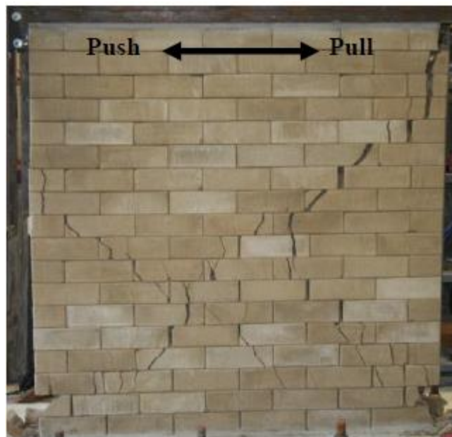
Figure 1: Wall 2 shear failure characterized by diagonal cracking and sliding displacement (Bland 2011)
