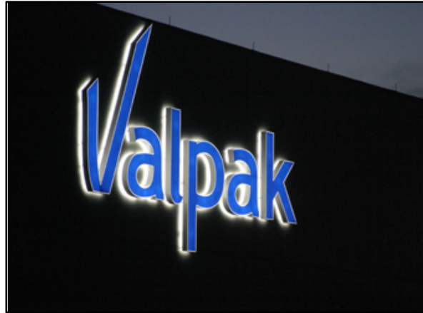
Figure 2.6: Internally Illuminated Sign ( www.intlsign.com )
