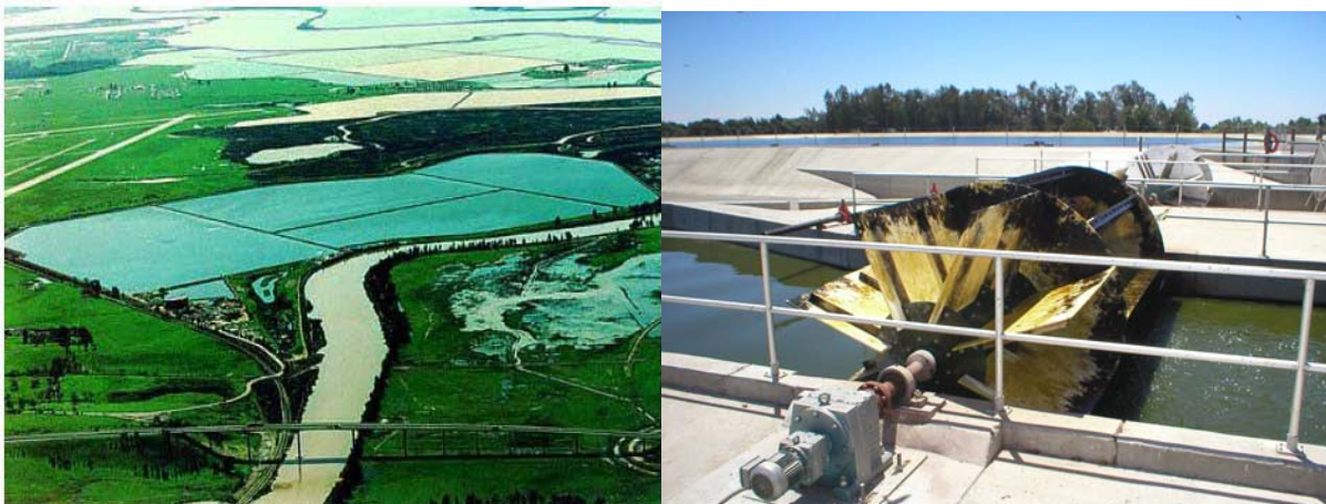
Figure 2.5 and Figure 2.6 Municipal wastewater treatment facilities.
