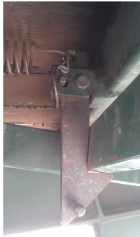
Figure 56. Ramp retaining bracket and linch pin.
