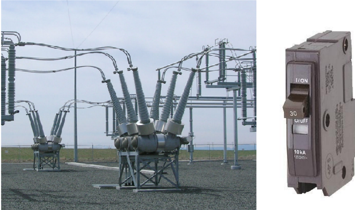
Figure 1-5: High voltage SF-6 Circuit Breaker (left) and low voltage miniature circuit breaker (right)
