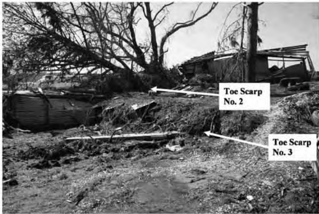
Fig. 6. View of Toe Scarp Nos. 2 and 3 at the inboard edge of the lateral translational failure at the 17th Street drainage canal
