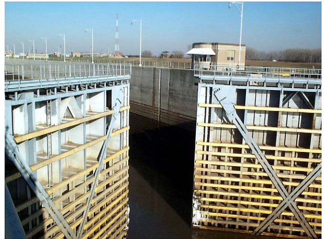
Fig. 12. Photograph of the miter gate on Lock and Dam 27 [8].
