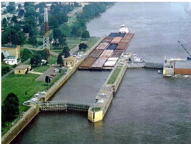
Fig. 2. Photograph of Lock and Dam 12 [27].
