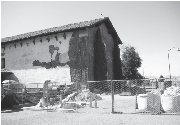
Figure 3 Repairs at San Miguel Mission, California.
