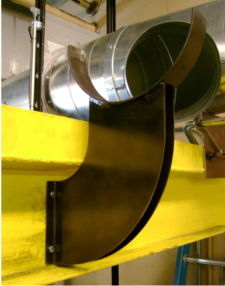
Figure 15. Beam bracket.
