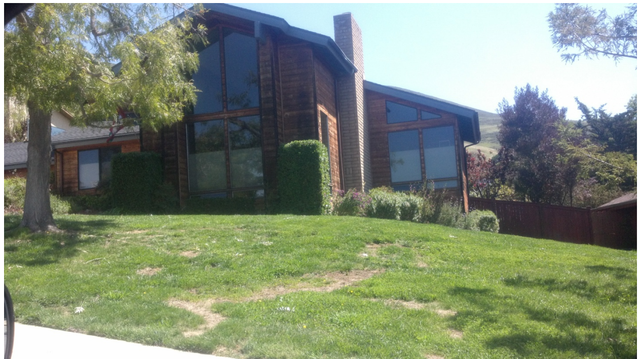
Figure 30. Older construction home with wood siding
