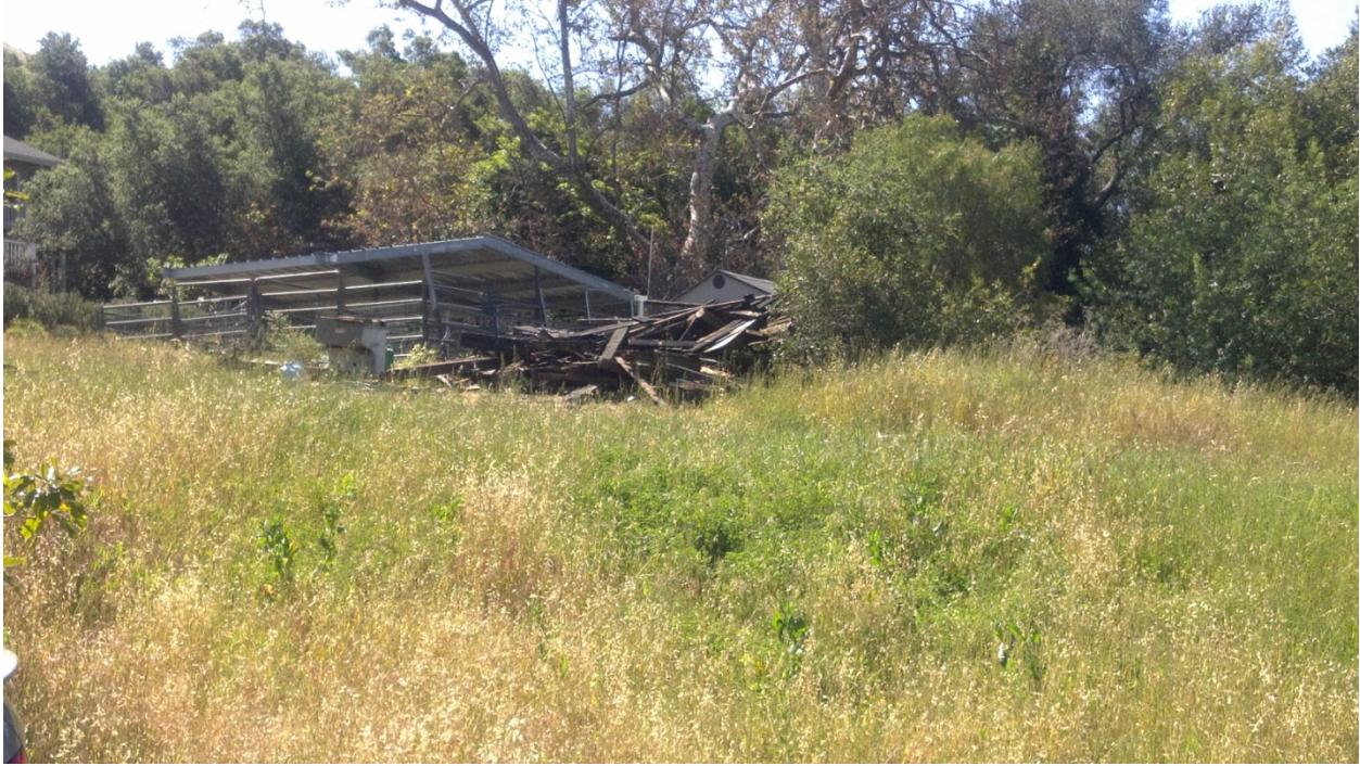
Figure 23. Woodpile on Andrew St. in a residents front yard
