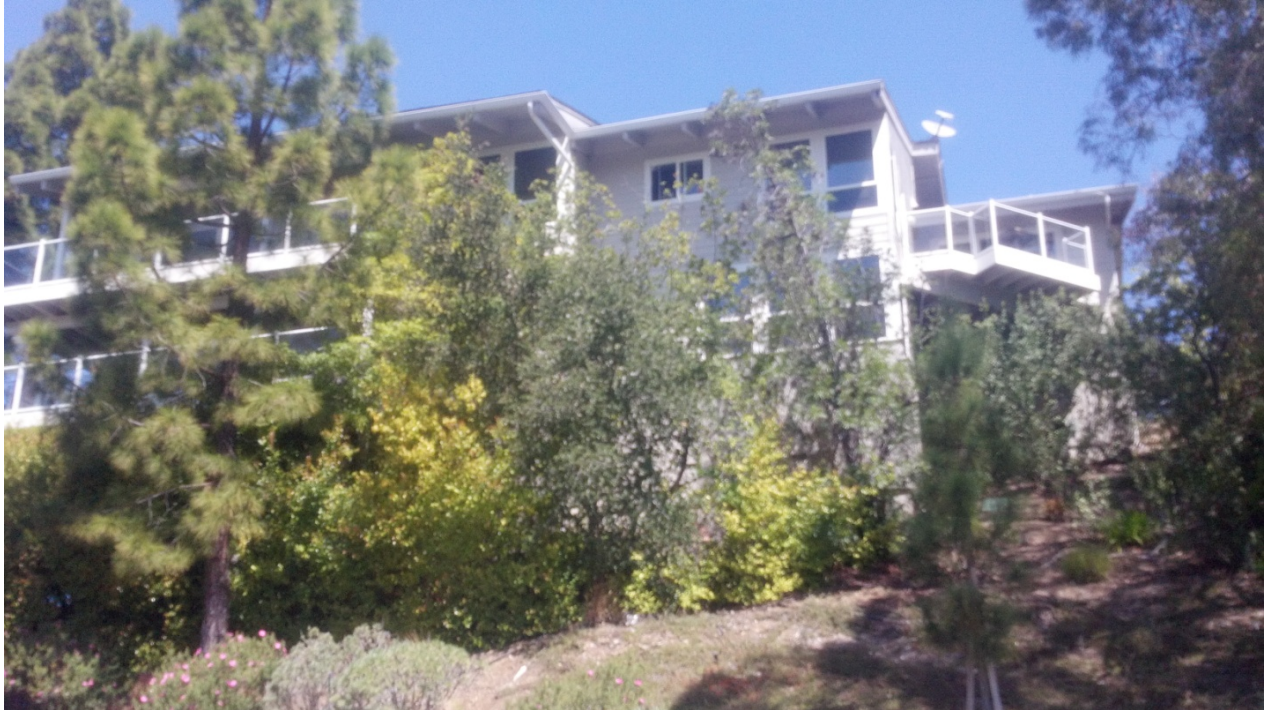
Figure 29. A house with flammable vegetation near the home and underneath the balconies
