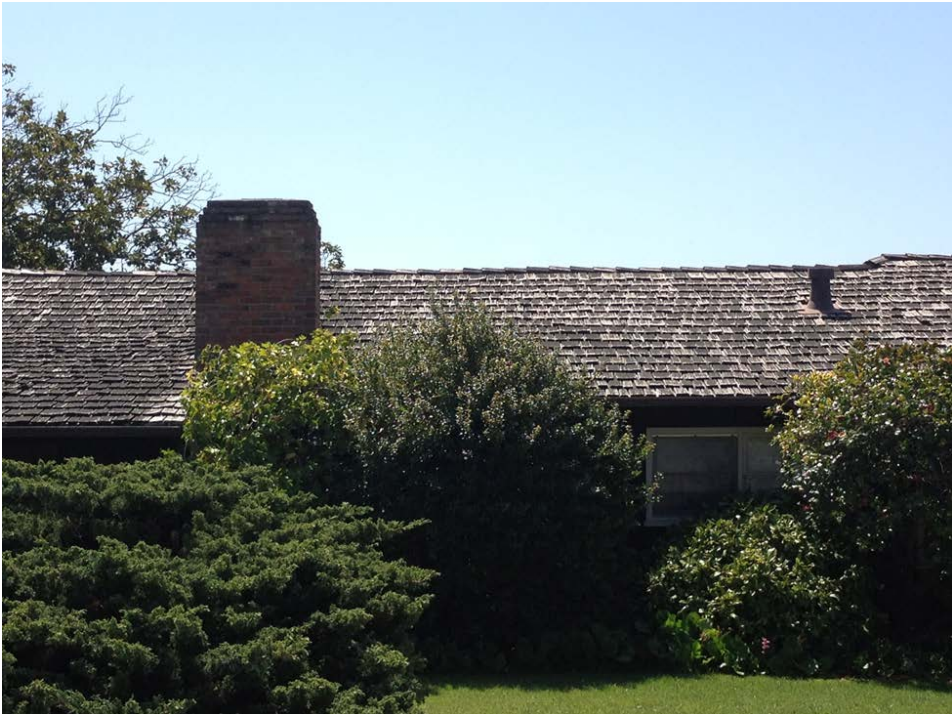
Figure 18. Example of wood shake shingle roof
