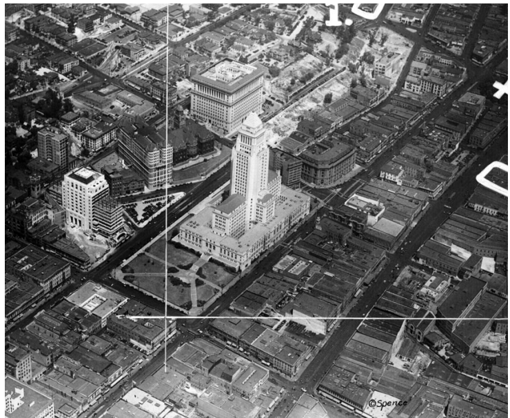
Figure 5.4. Aerial view of the Civic Center showing the completed City Hall and the California State Building under construction, August 22, 1931 (The Examiner)
