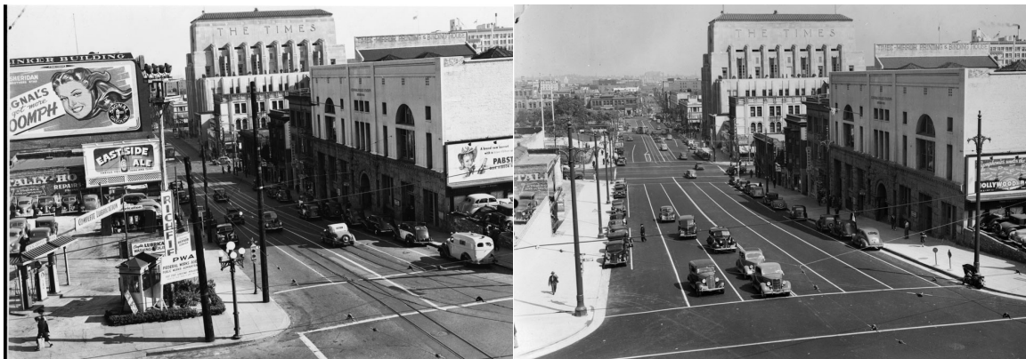
Figure 5.9. (Left) Looking east along 1st Street from Hill Street prior to widening (CHS)
