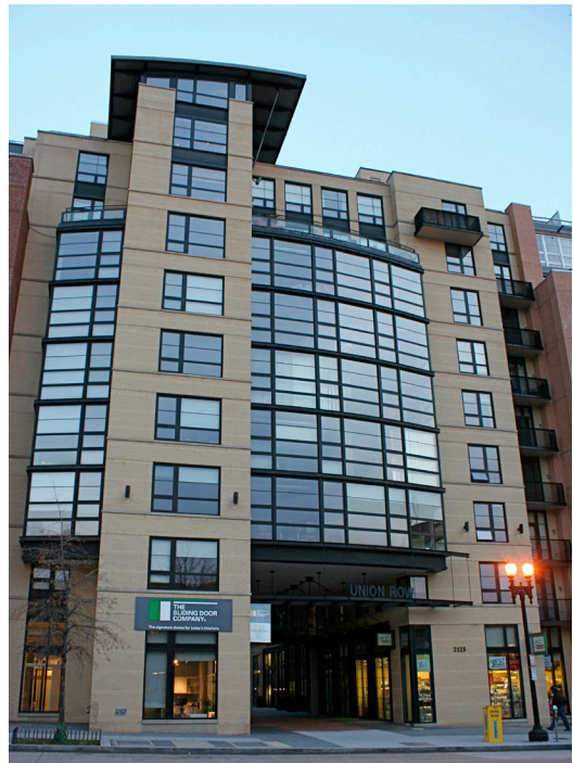
Figures 9.14 & 9.15. Facade differentiation, The Flats , Union Row, Washington, DC
