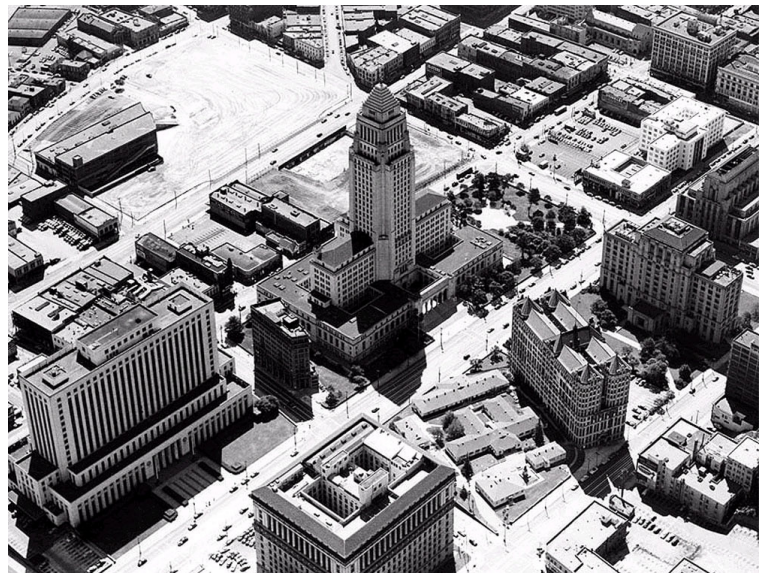
Figure 5.13. Aerial view looking southwest at the Civic Center showing land cleared for construction of the LAPD Headquarters
