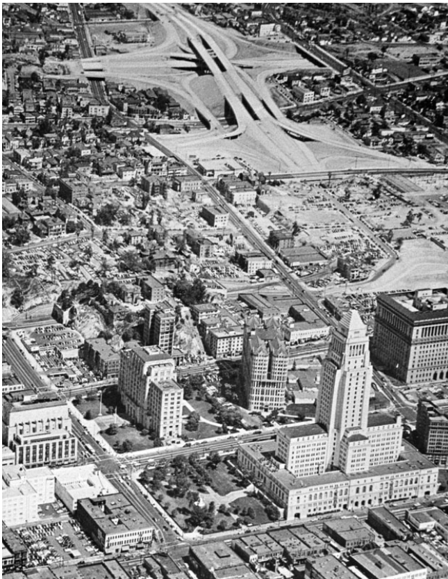
Figure 5.11. Aerial view of the four level interchange under construction (Los Angeles Public Library)
