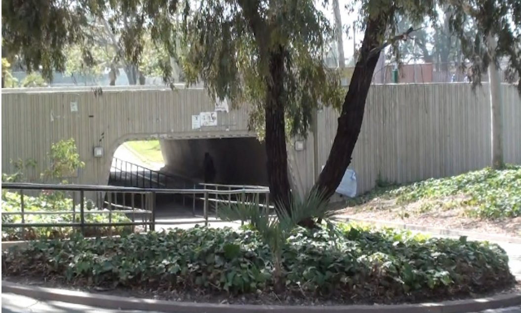
Figure 46. Underpass for Bicycle Path #1 – Santa Barbara, California
