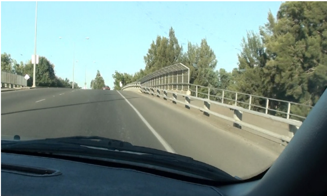
Figure 48. Bicycle Lane on Highway Bridge – Davis, California
