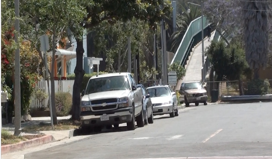
Figure 41. Pedestrian Overpass across US 101 – Santa Barbara, California
