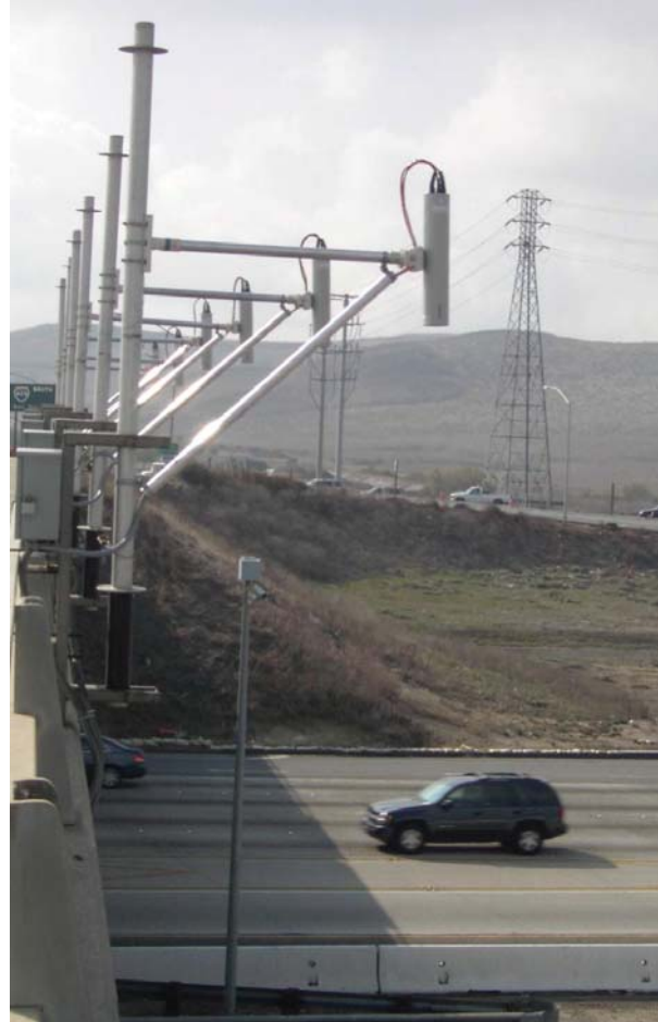
Figure 2. Down-looking video cameras above each lane.
