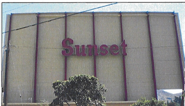
Figure 1.1 // Existing Drive-In Screen
