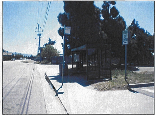
Figure 2.1 // Existing Bus Stop on Prado Road
