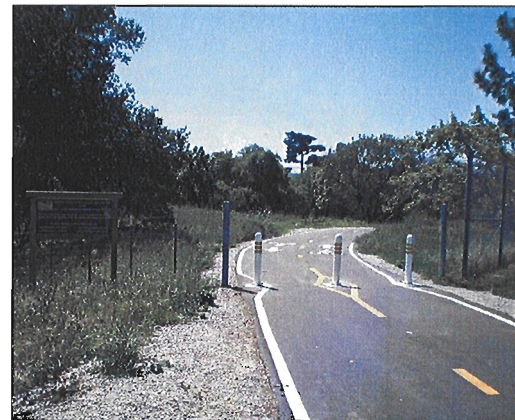
Figure 9.7// Existing Bob Jones Trail
