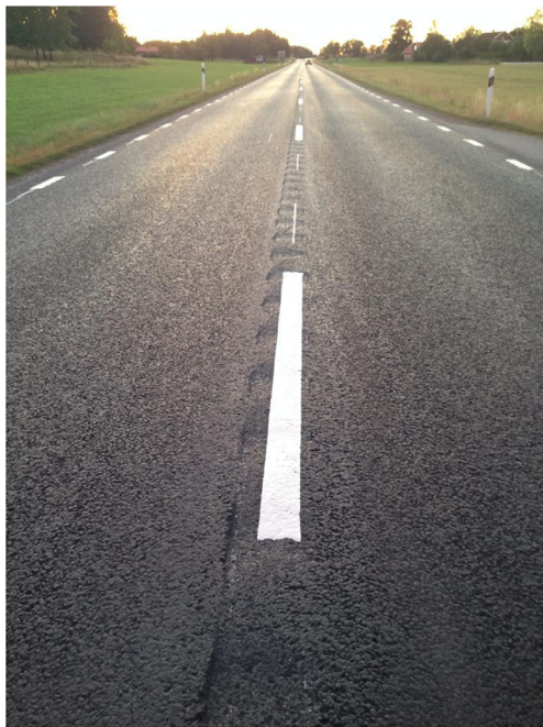
Fig. 1 Example of road with centreline milled rumble strips
