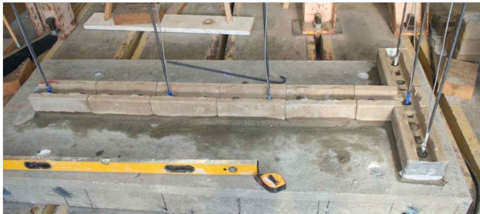
Figure 4-9: W5 after the first course was laid.
