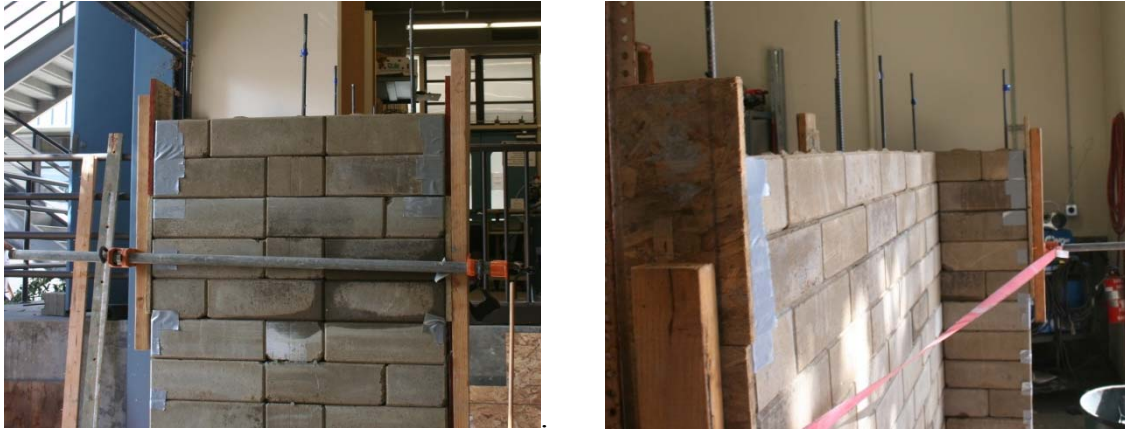
Figure 4-14: Courses 17 and 18 in the flange (left) and web (right) of W5
