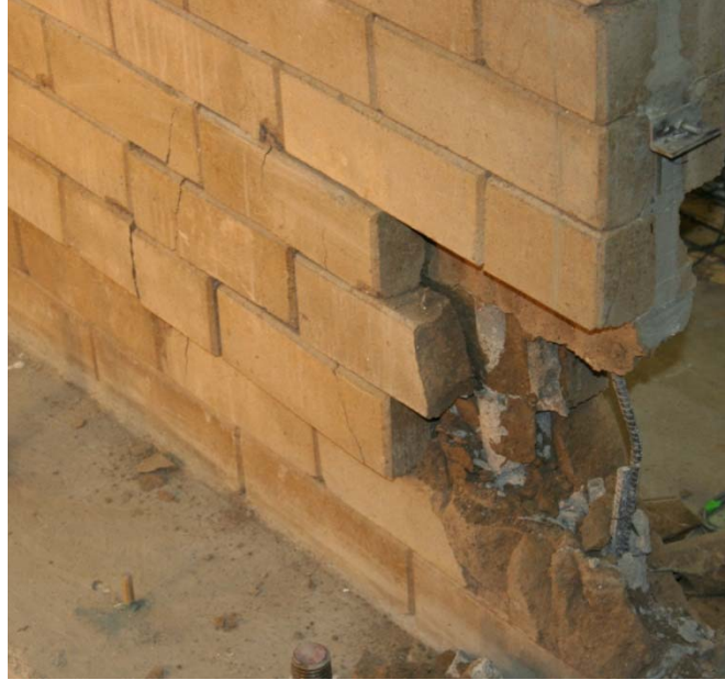
Figure 6-39: External spalling of ICEBs at the web toe of W5.
