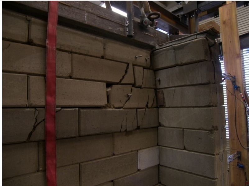
Figure 6-19: Compression failure at the intersection of the web and flange
