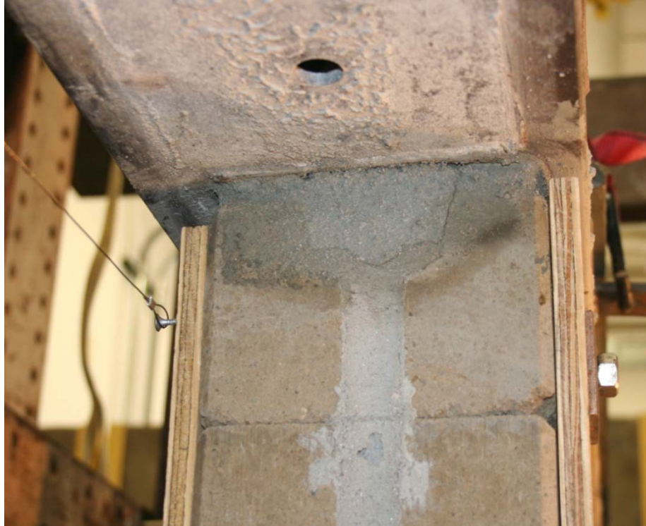
Figure 6-8: W4 cracking around the grout channel and the loading beam
