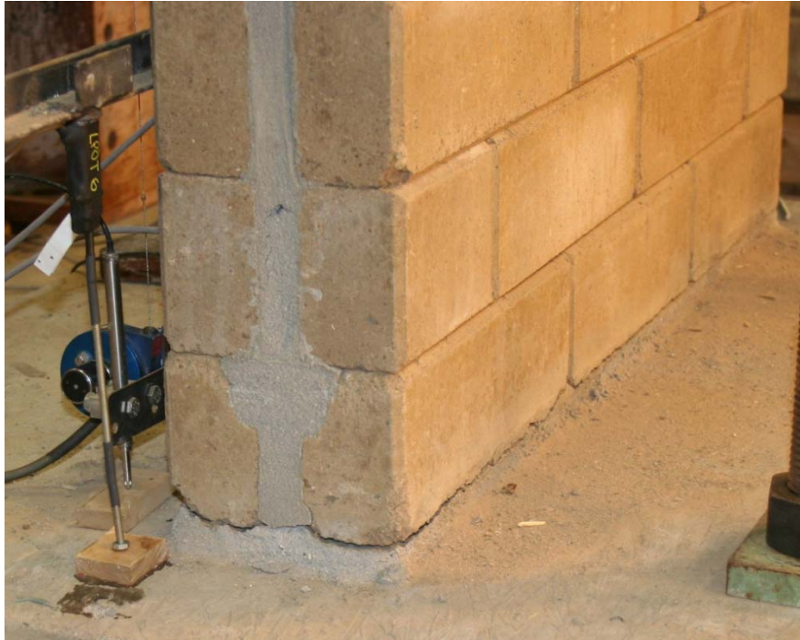
Figure 6-7: Cracking around the base of W4
