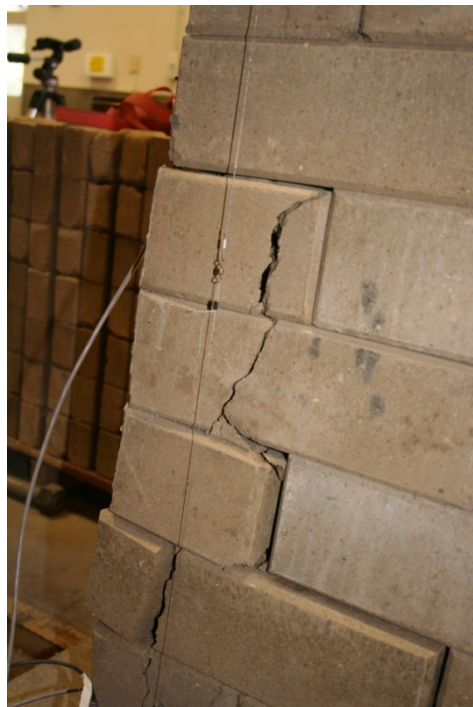
Figure 6-35: W5 cracking around the bottom toe of the web
