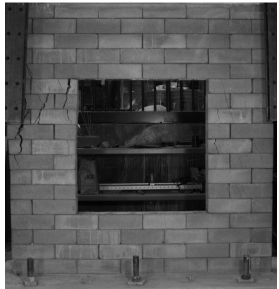
Figure 6-54: Cracking pattern of W6 following Cycle 22
