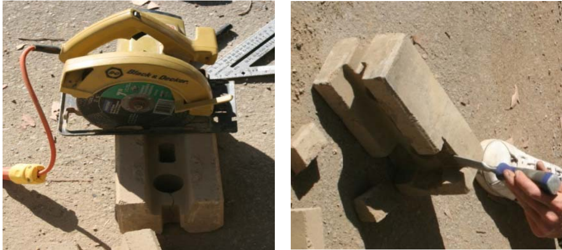
Figure 4-8: Modification of end blocks for reinforcement
