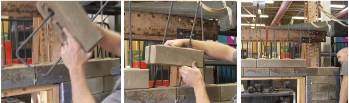
Figure 4-22: Setting the shear reinforcement for the lintel of W6
