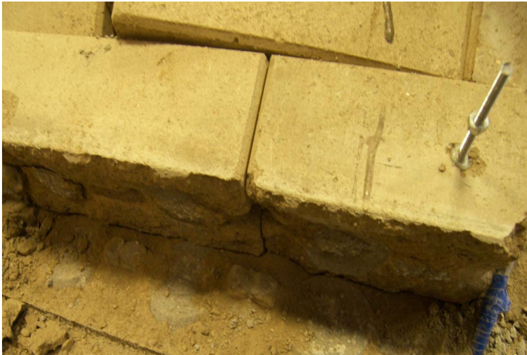
Figure 6-9: Shearing between the bottom courses of W4 and the mortar in the footing
