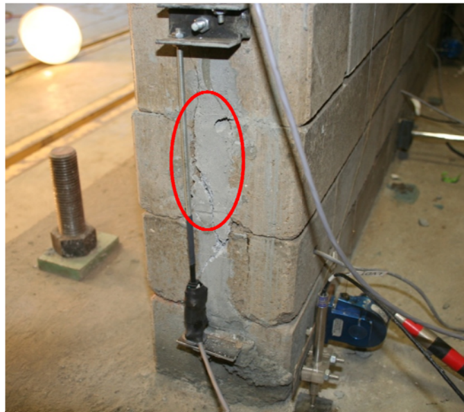
Figure 6-30: Tension cracks at the base of the toe of W5 web
