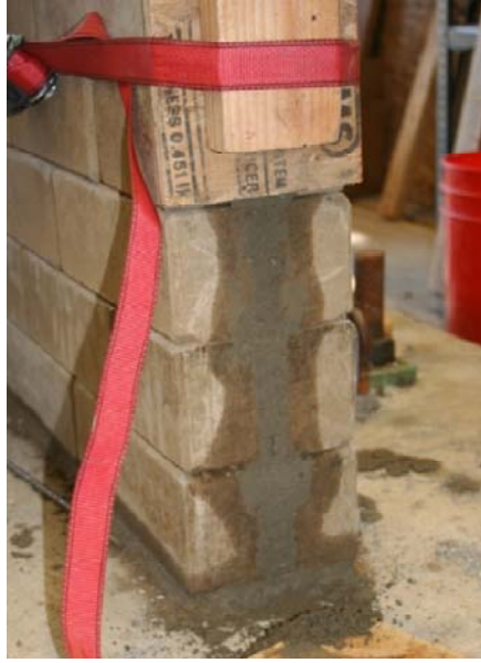
Figure 4-6: Plywood confinements for grout keys
