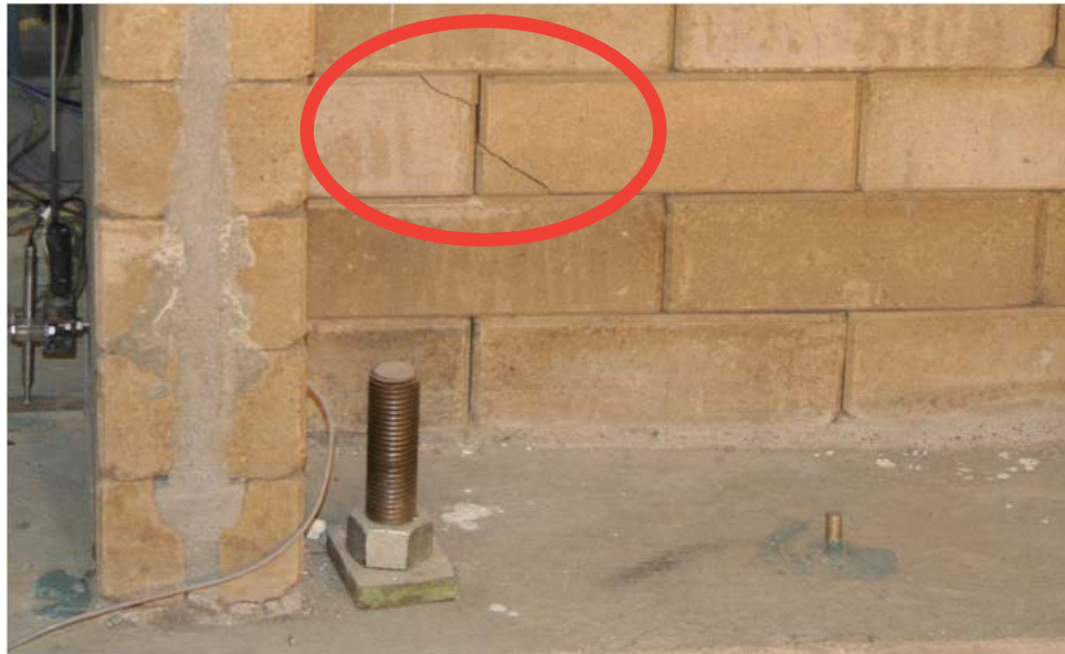
Figure 6-27: Crack in the W5 at maximum displacement of cycle 8
