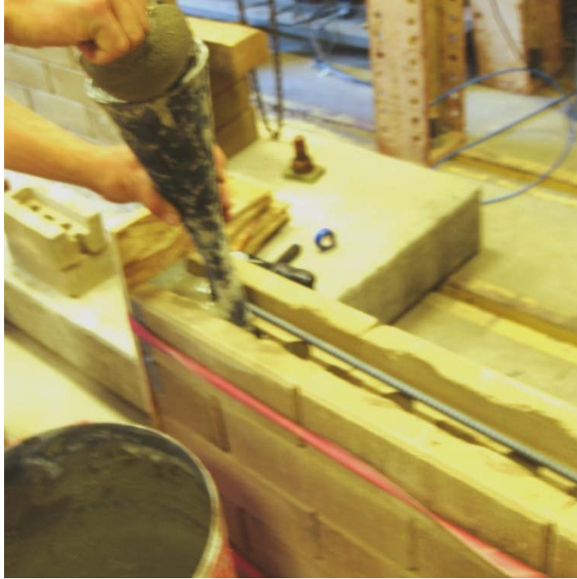
Figure 4-19: Courses 1-4 of W6 being grouted
