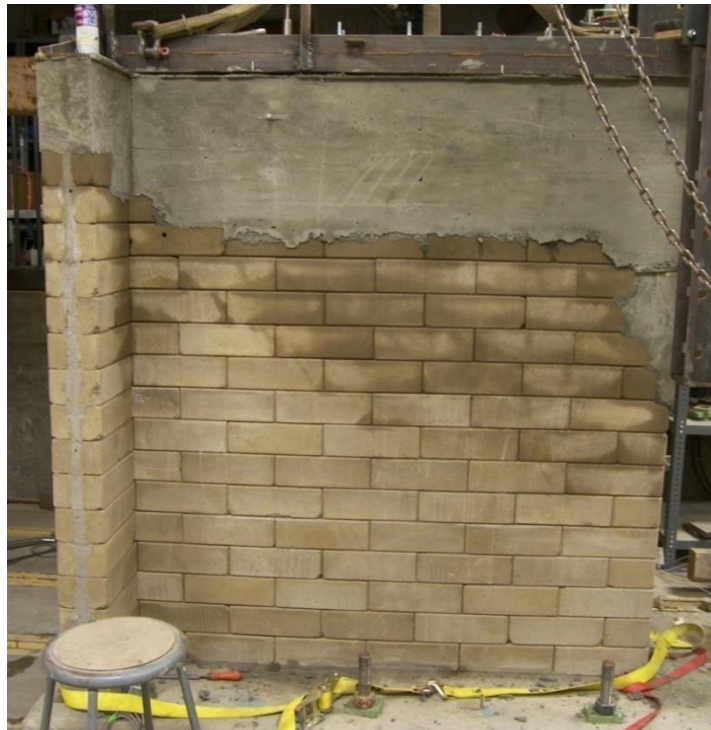
Figure 6-23: Web of W5 after removal of the reinforced concrete formwork
