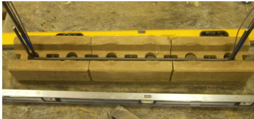
Figure 4-4: Rebar Anchored Footing of W4
