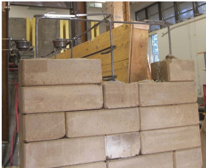
Figure 6-22: Repair of the flange of W5 before reinforced concrete was cast
