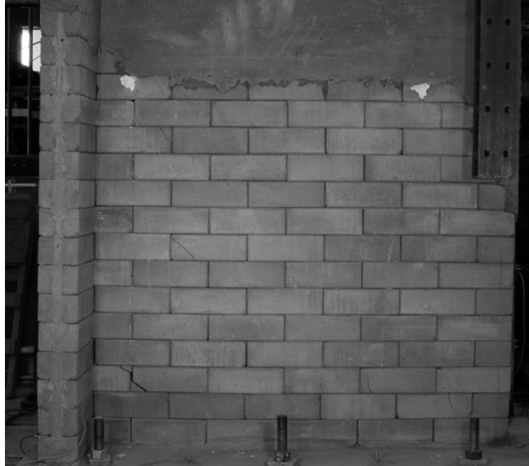
Figure 6-33: Cracking of W5 web at zero displacement after Cycle 16
