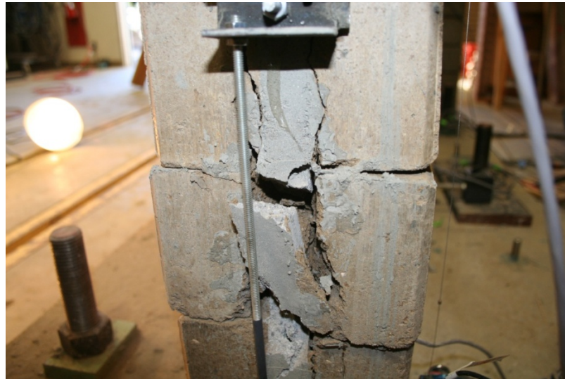
Figure 6-32: Spalling of the outer grout channel of the W5 web during Cycle 16
