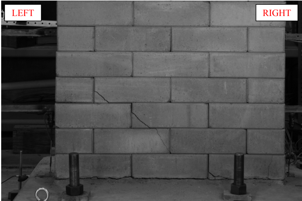
Figure 6-10: Shear cracking along the bottom of W4
