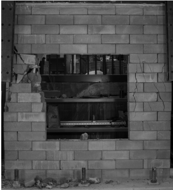
Figure 6-55: Damage in W6 following Cycle 24
