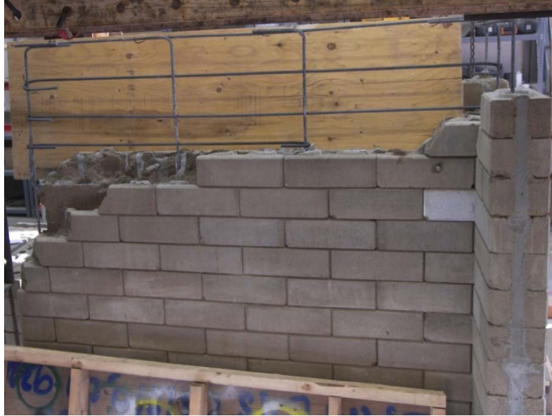
Figure 6-21: Repair of the web of W5 before reinforced concrete was cast
