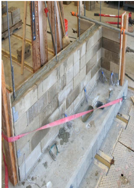
Figure 4-13: Courses 1 through 5 of W5 after grouting,
