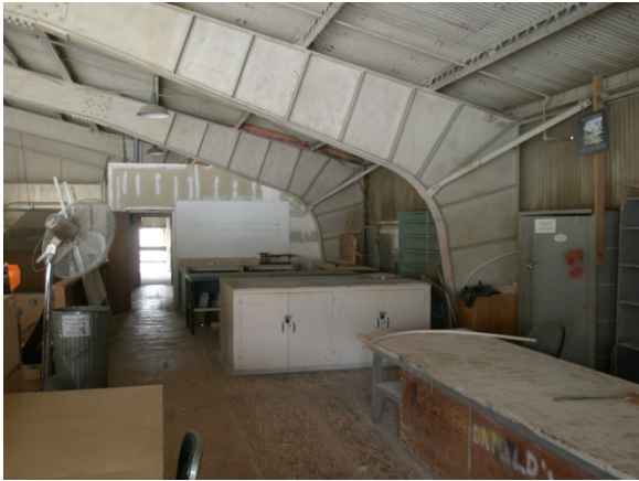
Figure 12 - Manufacturing Floor View 1
