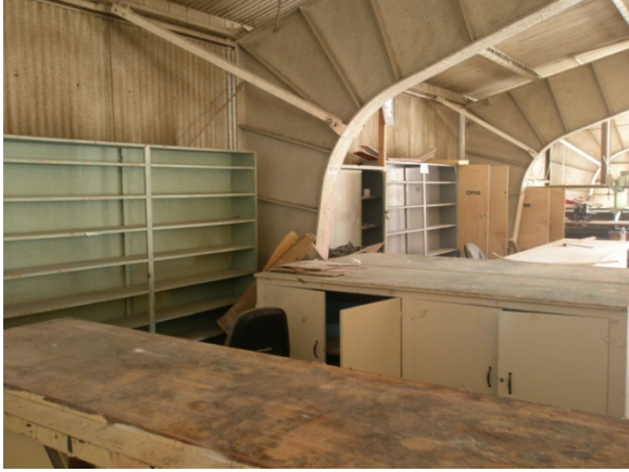
Figure 14 - Manufacturing Floor View 2
