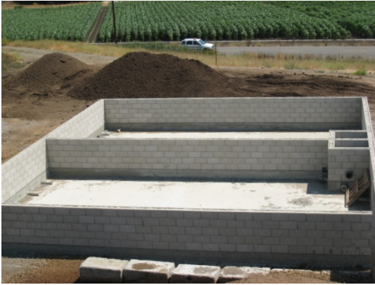
Figure C.1. Completed, empty basins. View from solids separation screen.
