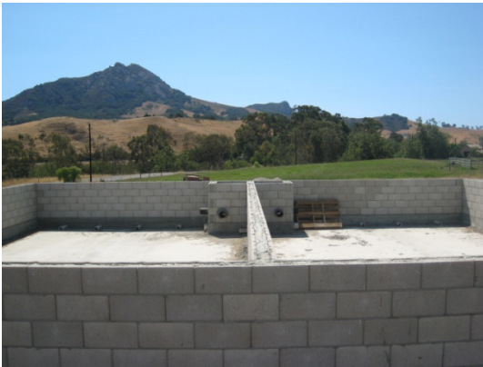
Figure C.2. View of completed basins from ground level.
