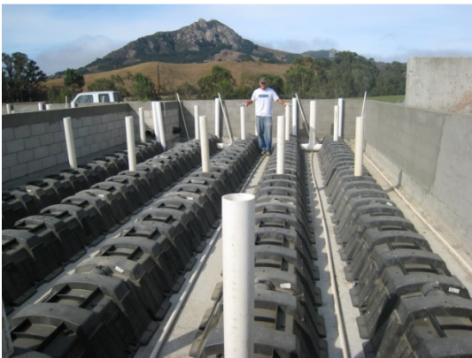
Figure C.6. Completed leach field chamber installation. Three standpipes in each chamber row.
