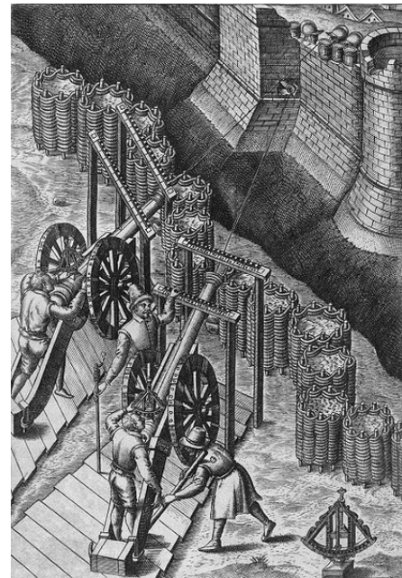
Figure B - Gabions used for 16th-Century artillery protection
